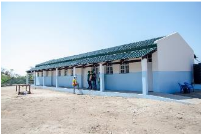
Construction of the Mutua Primary School in progress, in August 2021. Eight new primary schools on-going in Chibabava and Dondo districts.
