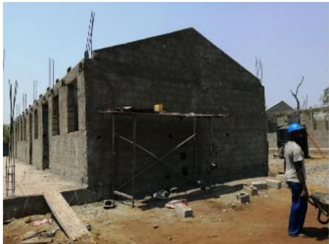
Girome Primary School in progress, in September 2021.
