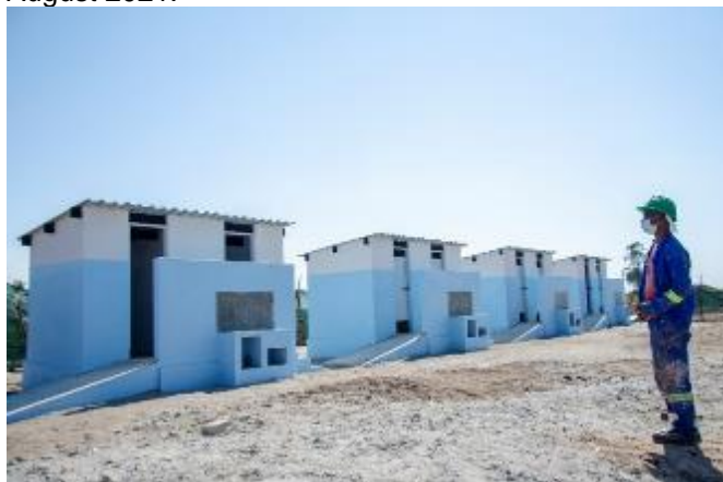
Latrines built following the BBB standards, in the primary school of the Mutua resettlement neighborhood, Dondo, in August 2021.
