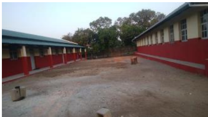
Chipinde Primary School in September 2021.
