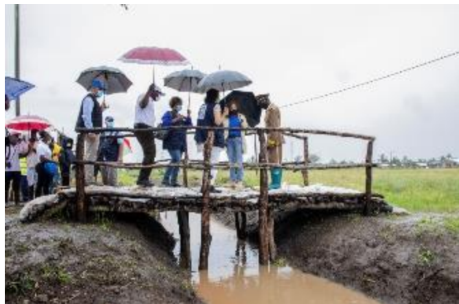
Small bridge rehabilitated through cash-for-work, in Buzi-Sede, Buzi district, in December 2020.
