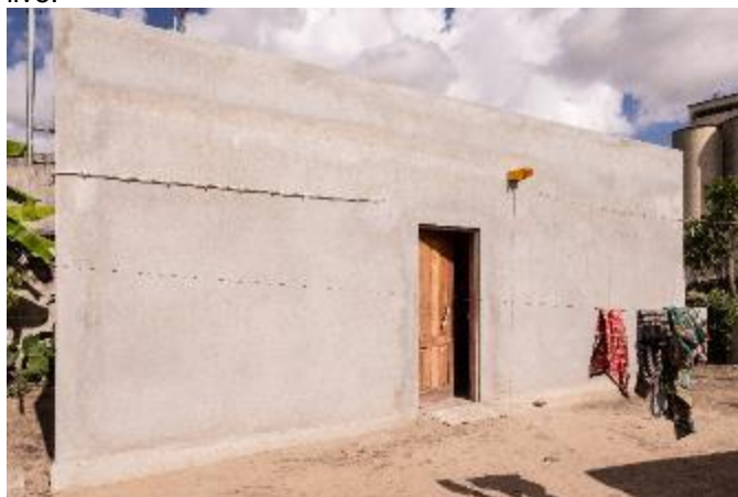
Ms. Nhawa Domingos's house after rehabilitation, following the BBB standards, in May 2021, in the peri-urban area of Beira city where hardly affected population live.
