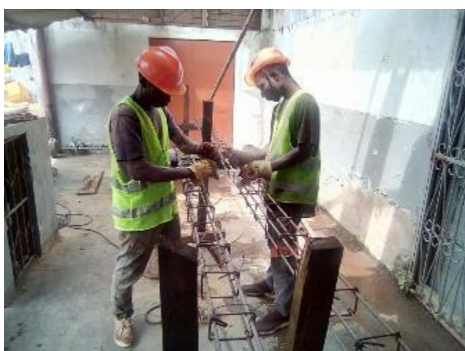
Preparation of beam for a house rehabilitation, in Mandruzi, in September 2021.
