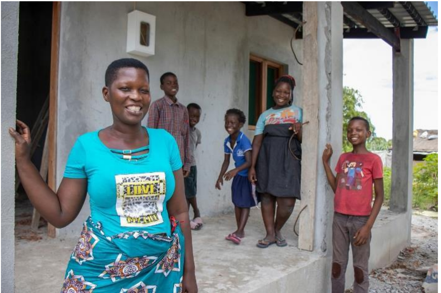
Cecília Chata Valentim and her children in front of the new house under construction. Photo by UNDP.
