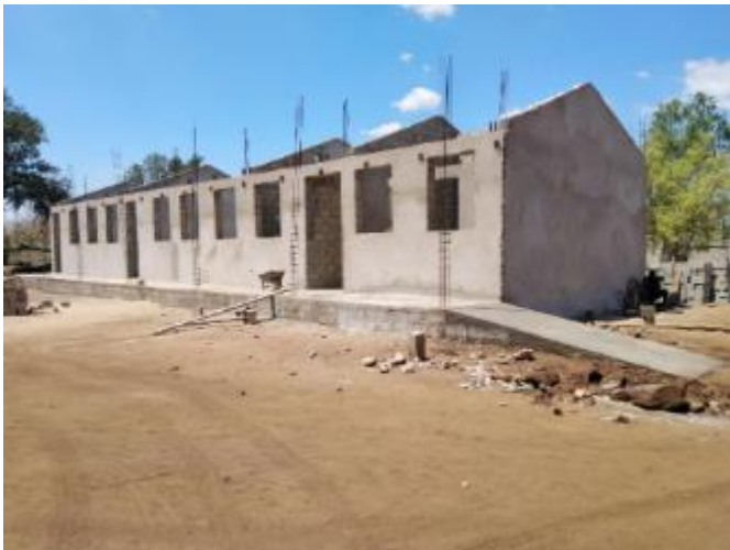
Construction of the Heua Primary School in progress, in September 2021.
