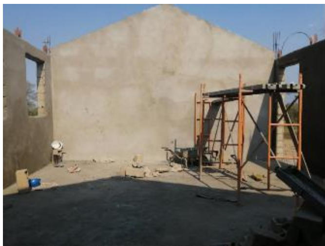
Armando Emilio Guebuza Primary School in progress, in September 2021.
